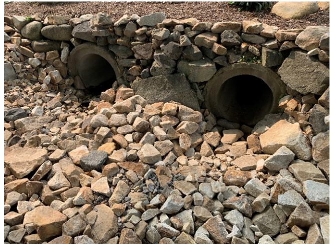
64 Gundalow - 2 (Drainage Course)
