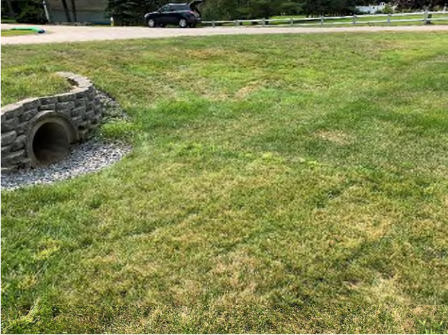
29 Gundalow - 1 (Drainage Area)
