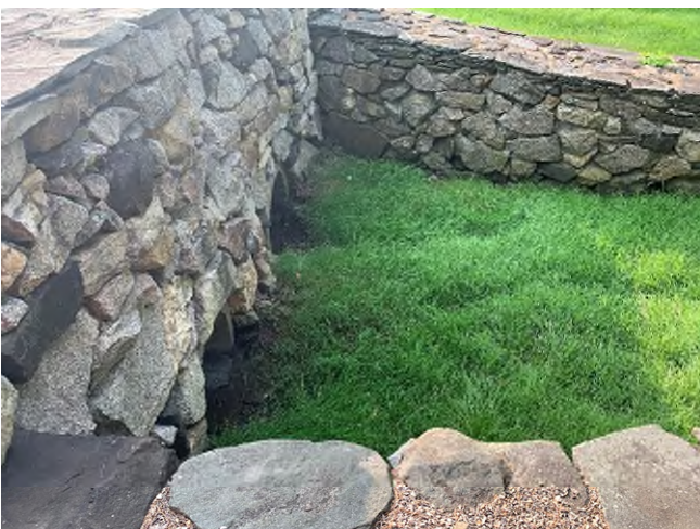
4 Brickyard Circle - 1 (Drainage Course)
