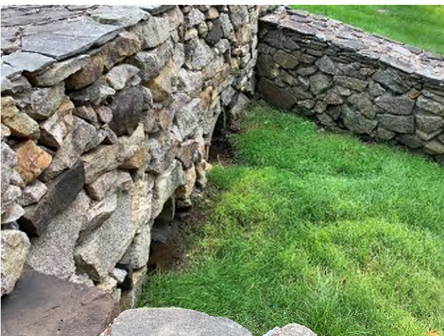
4 Brickyard Circle - 1 (Drainage Course)
