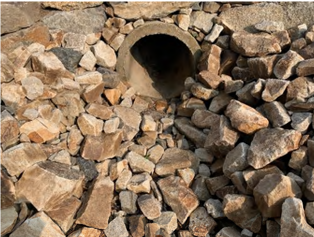
64 Gundalow - 1 (Drainage Course)
