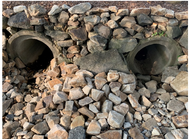
64 Gundalow - 2 (Drainage Course)
