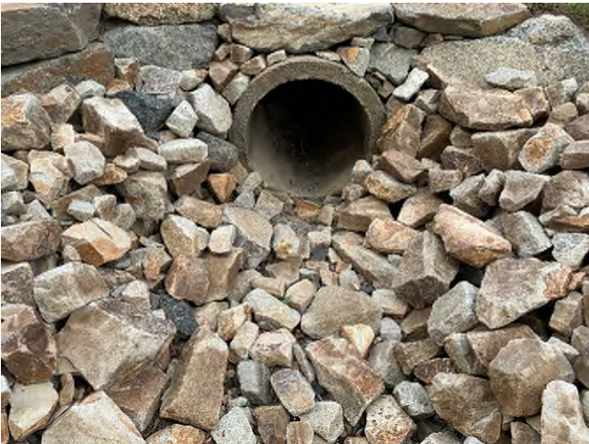
64 Gundalow - 1 (Drainage Course)
