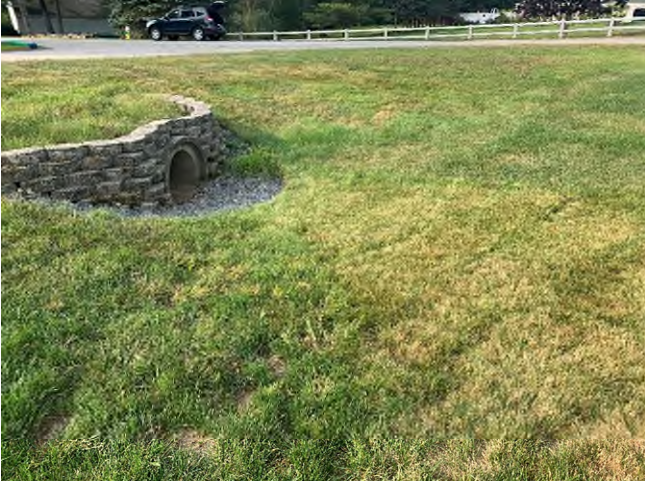
29 Gundalow - 1 (Drainage Area)
